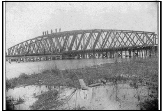
The Solberg Point draw bridge was reconstructed during the winter of 1893-1894. Men posed for a photograph on the newly completed bridge, April 1894.
