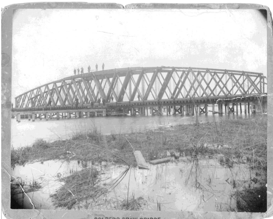
Solberg Draw Bridge in 1894. Built for Minneapolis & St. Louis Railway in 1881 between Excelsior and St. Alban's bays.
